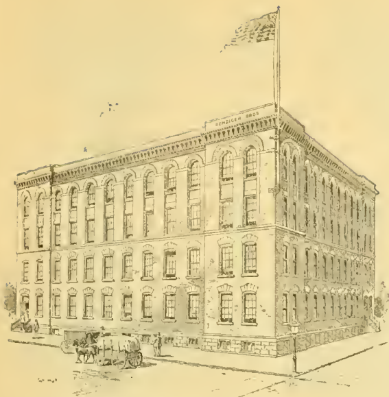
BENZIGER BROTHERS' FACTORY, De Kalb Avenue and Rockwell Place, Brooklyn, N. Y.
